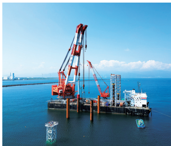
Fig. 15 Installation of piles at the site
