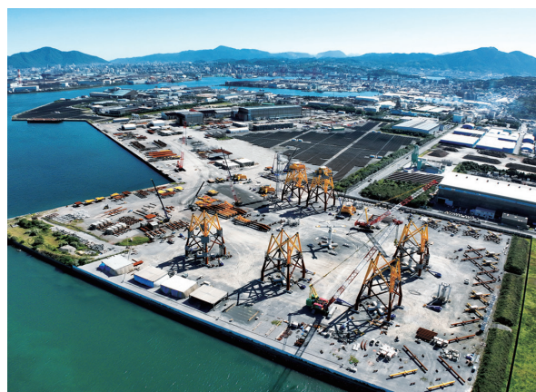
Fig. 16 Jacket structure under construction at Nippon Steel Steel Structure Co., Ltd.
