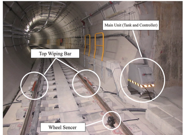
図8 摩擦調整材塗布装置 Application equipment of friction modifier
