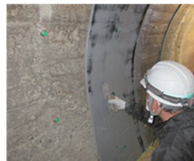
写真5 CFSS施工状況 Adhesion work of CFSS
