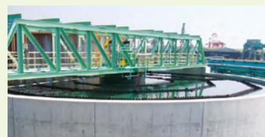
Undissolved residue from rainwater is coagulated and settled, and eliminated.
