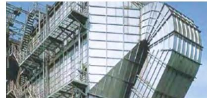
Dust generated in the burning process is collected by two types of dust collectors (electric or with bag filter), depending on the characteristics of the dust (i.e., particle size distribution, emission gas concentration.)
