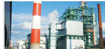
The dry desulfurization and denitrification methods, using active coke, enables SOx and NOx in emission gas to be eliminated.
