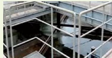
Floating oil is removed by tiny bubbles formed by released air.
