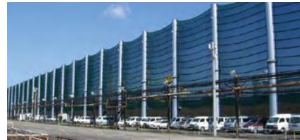
A windbreak net is installed to reduce the strength of wind and restrain the scattering of raw materials.
