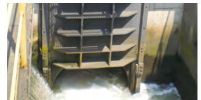
Water discharge flow is shut in case of trouble.
