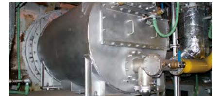
Burners featuring reduced levels of NOx generation and outstanding fuel savings have been installed.
