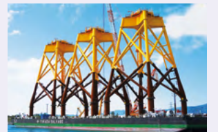
Jacket-type foundation to support offshore wind turbines
