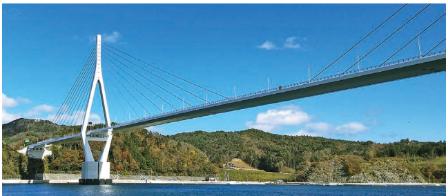
Kesennuma Bay Crossing Bridge
