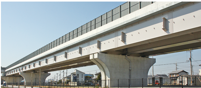
Higashi-Harima Nanboku Road (Mizuashi Shintsuji No. 5 Viaduct)
