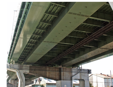
Hanshin Expressway Sambo Junction
