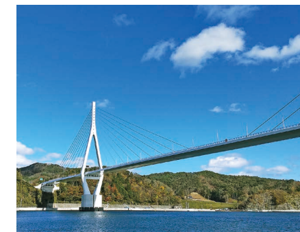
Kesennuma Bay Crossing Bridge
