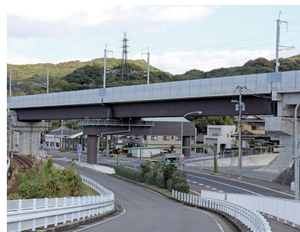
Uzu Viaduct Bridge (Nagasaki prefecture)
