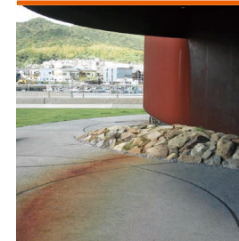
Discoloration due to rust in the shape of a flow or stream
