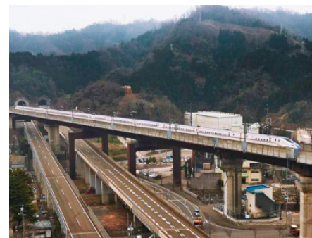
Hokuriku Shinkansen Hokurikudo Overbridge (Niigata Prefecture)
