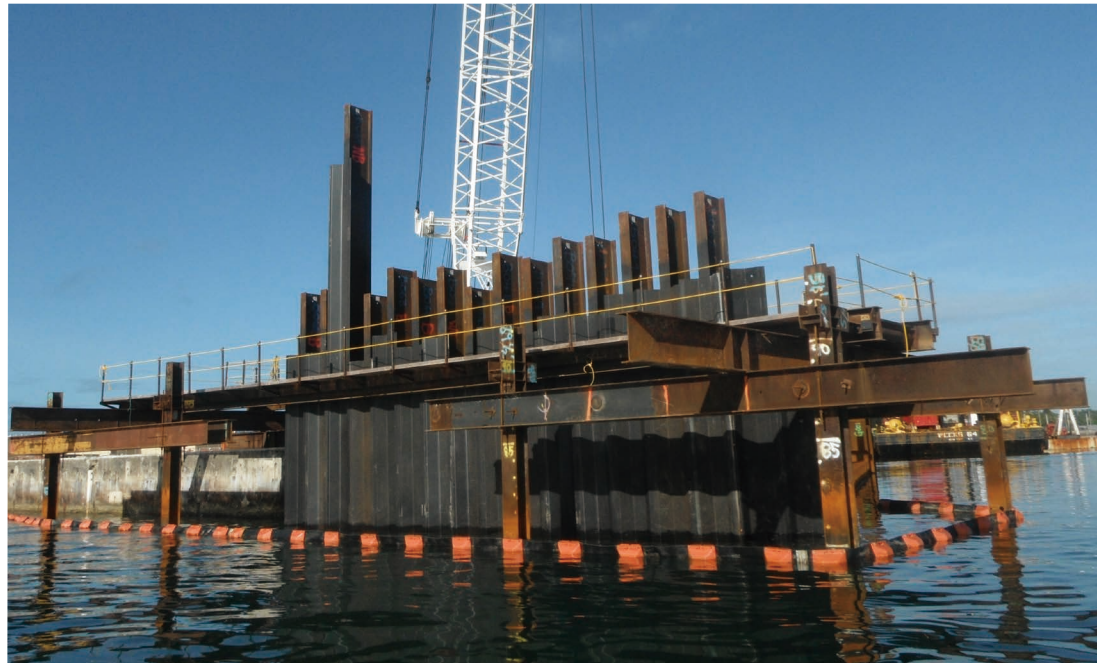
Hat+H Guam Apra Port refurbishment / USA
