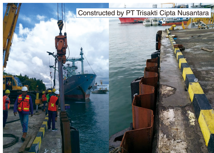
Hat-type Sheet pile Quay wall as port reinforcement in Benoa Port / Indonesia
