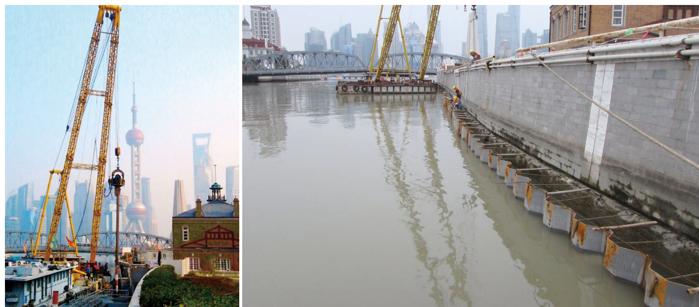
Hat-type Sheet Pile / China
