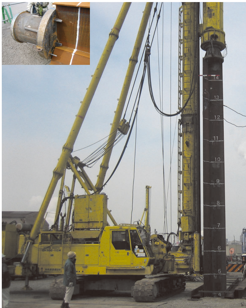
Driving of a Hat+H sheet pile
