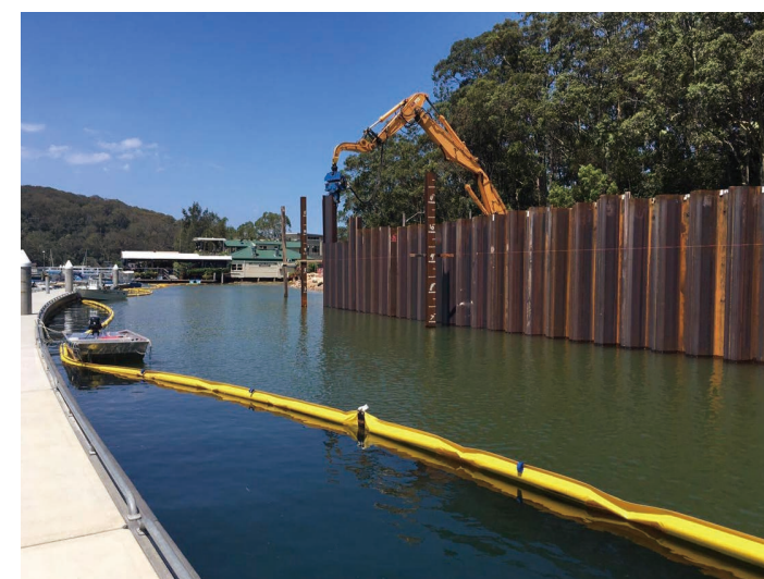
Hat-type Sheet Pile Church point seawall / Australia
