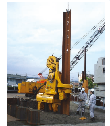
Pressing-in of U-type sheet pile
