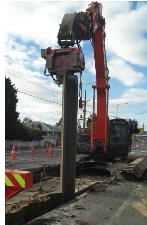
Driving of a Hat-type sheet pile
