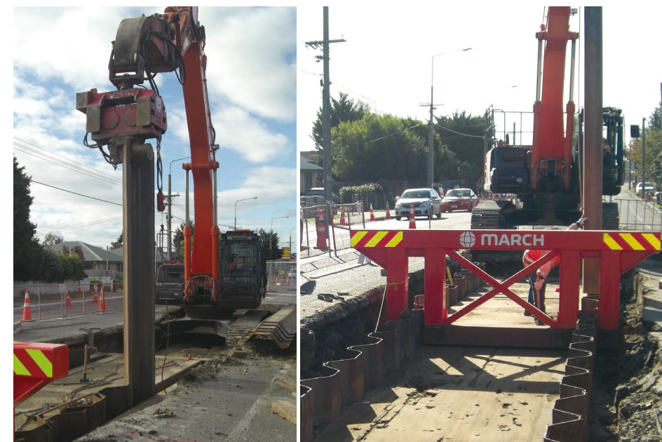
Hat-type Sheet Pile / New Zealand
