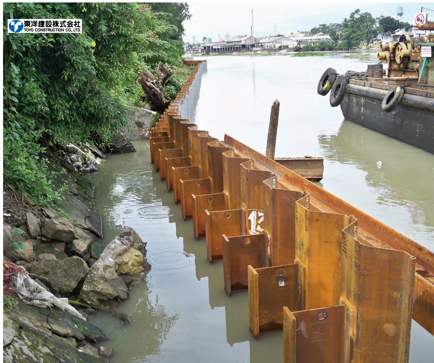
Hat+H Pasig-Marikina River Channel Improvement Project(Phase 3) / Philippine
