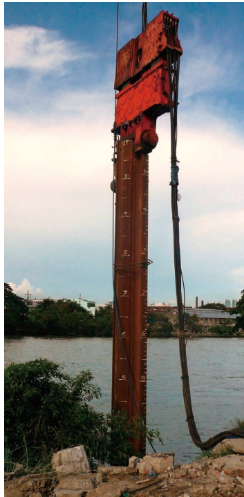
Driving of a Hat+H sheet pile
