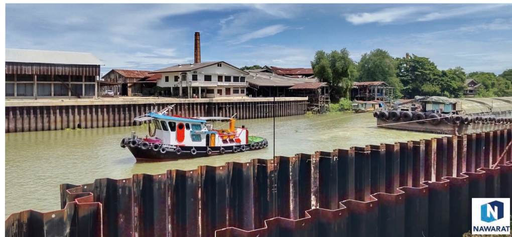
Hat-type Sheet pile River revetment / Thailand
