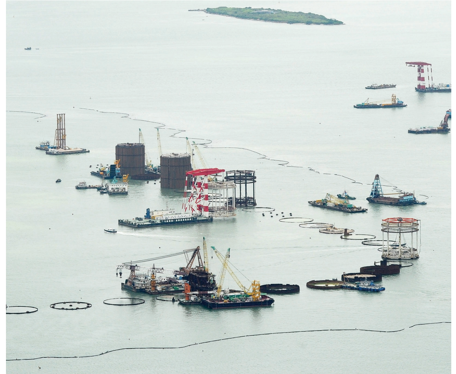
Steel Sheet Pile Cell (Straight web-type sheet pile) Hong Kong Macau Artificial Island / Hong Kong
