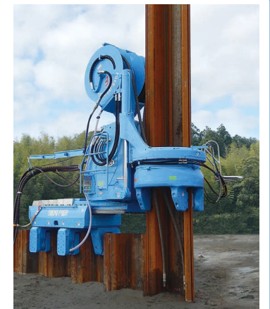
Pressing-in of Hat-type sheet pile
